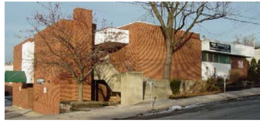
GIRD Systems Headquarters in Cincinnati, OH
